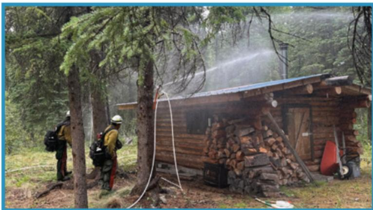
*Firefighters test a sprinkler system on a remote cabin while working on the Sinnott Fire north of Eagle in July 2024.*
